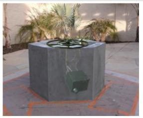
Remember to place the burner ring high enough over the valve to prevent overheating
